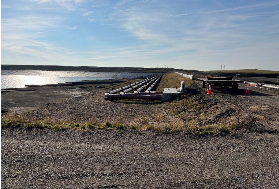
Photo 1 Bottom ash sluice piping, interior of west dike looking south. 11/5/2021
